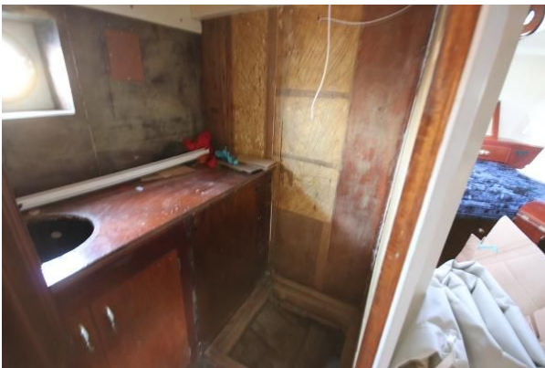
Gentleman's Yacht shower room incomplete
