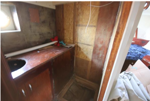
Gentleman's Yacht shower room incomplete
